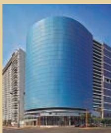
LIMA CENTRAL TOWER
